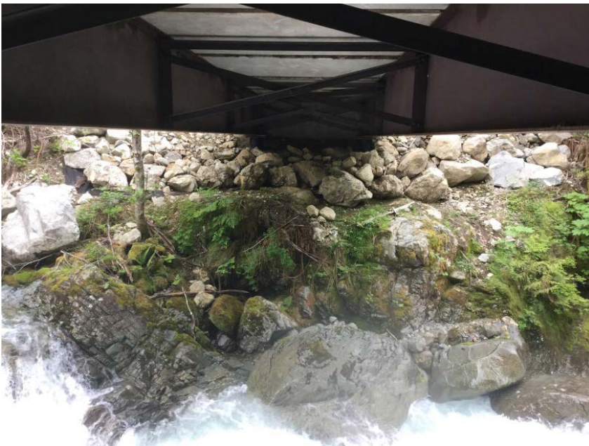
Left Bank Abutment when facing downstream
