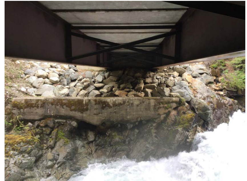
Right Bank Abutment when facing downstream
